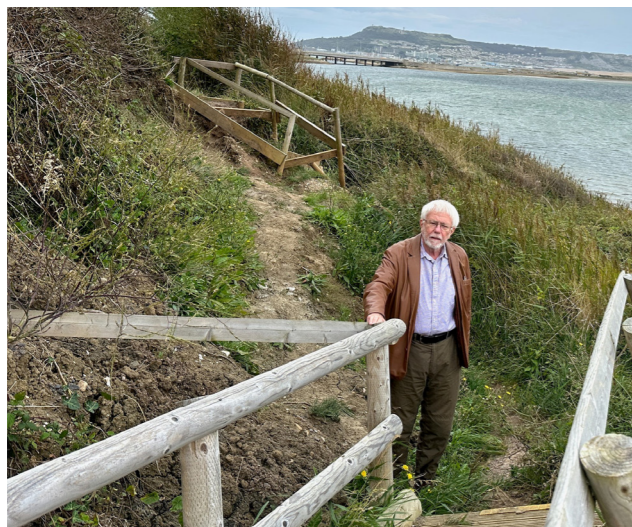
Brian at the collapsed steps in Wyke
